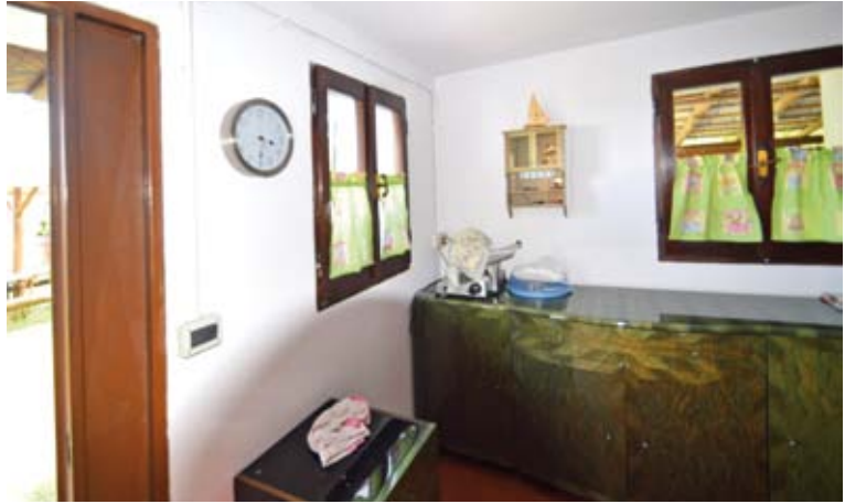
Wall maintenance with lime based paint
