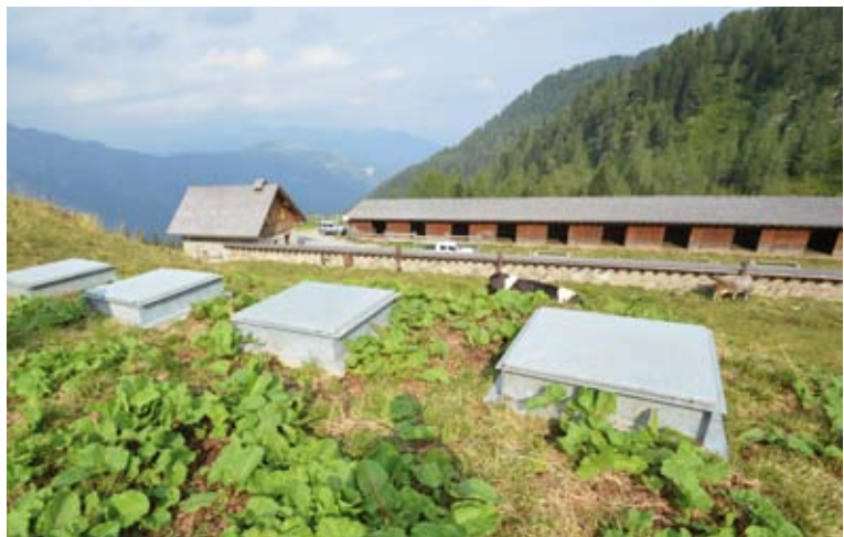
Adequate ground reservoir for water storage
